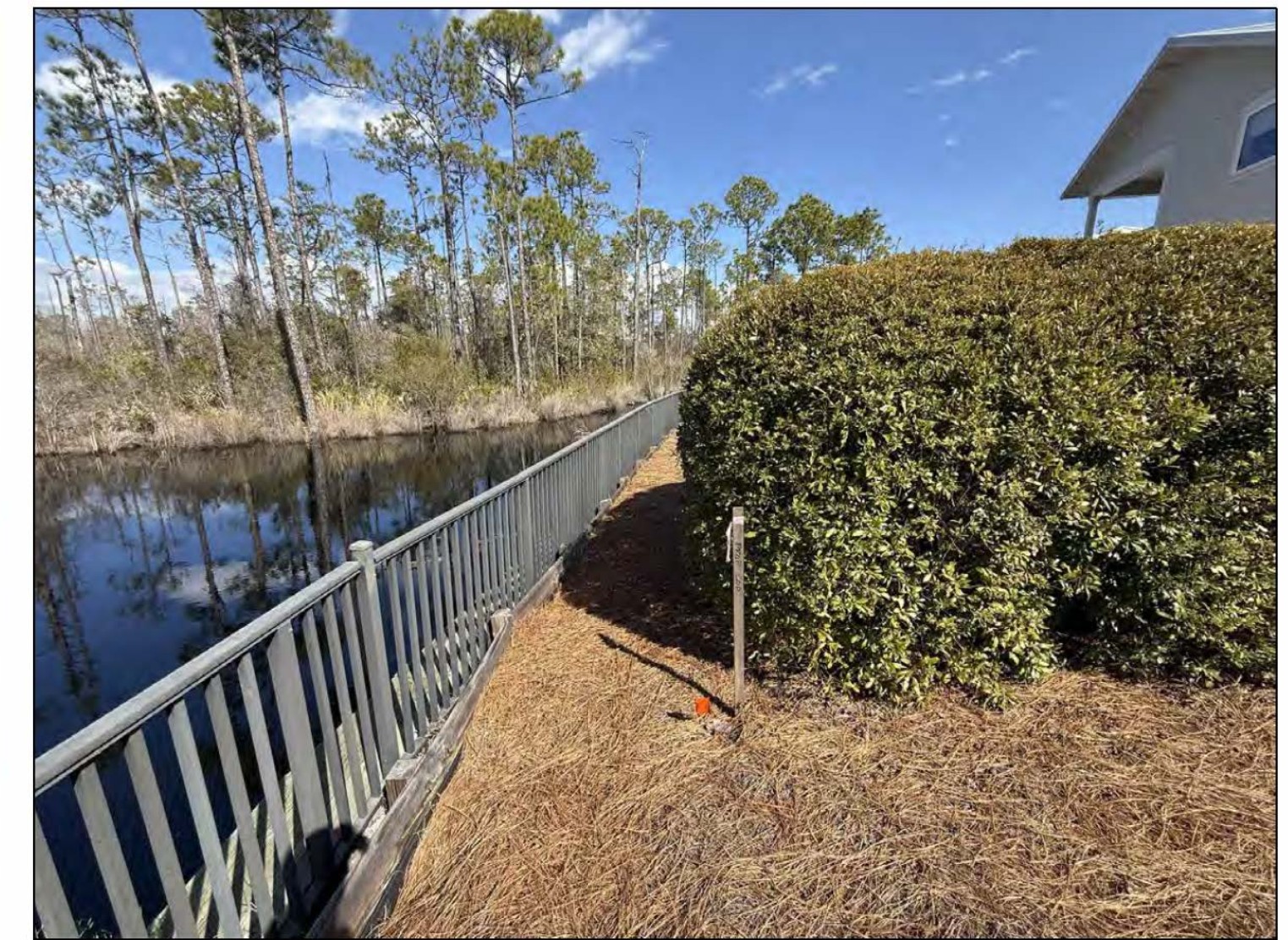
CDD FILL/WALL BEHIND LOT 259
