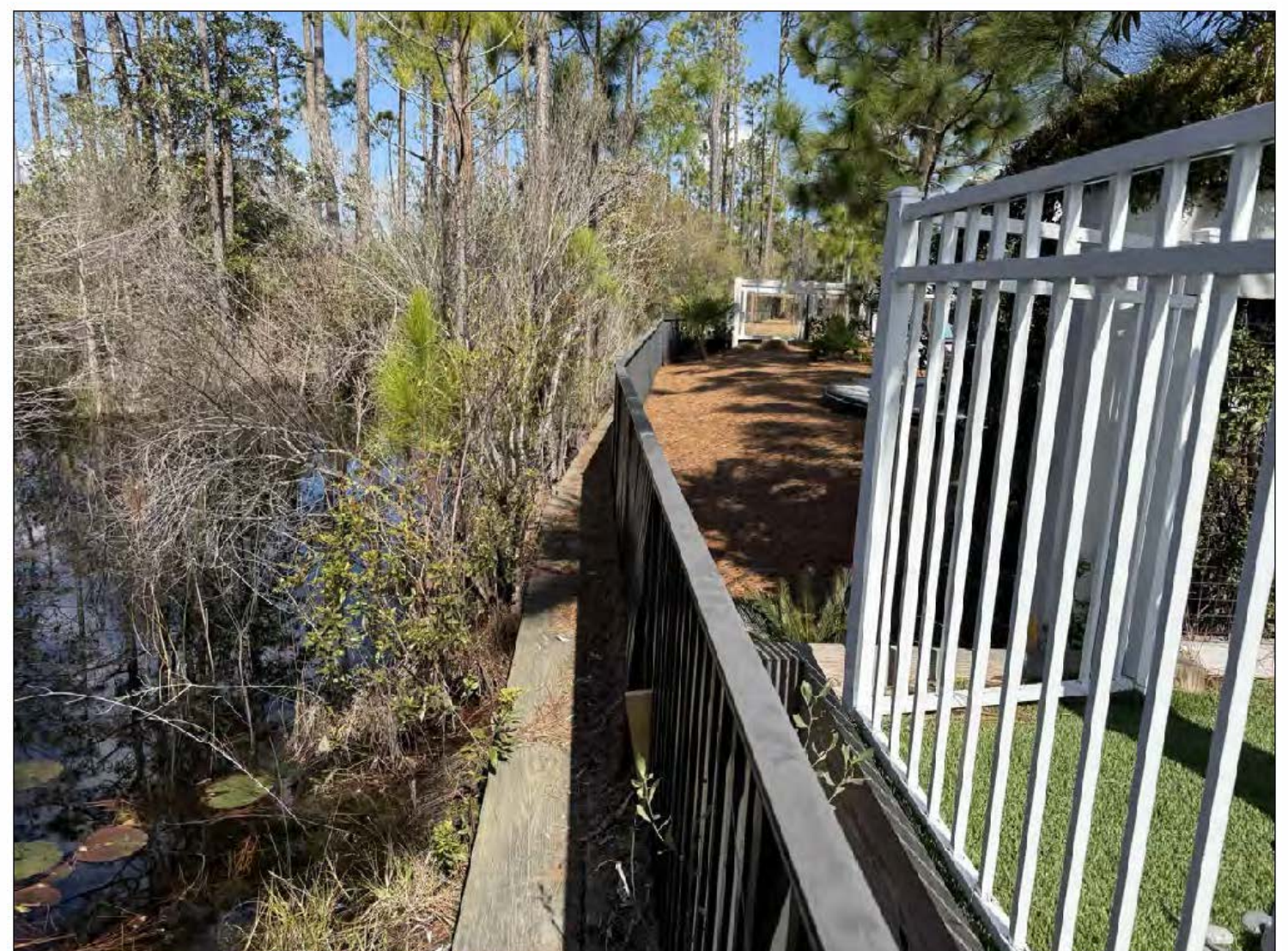
FENCE /WALL ENCROACHMENT ON LOT 254
