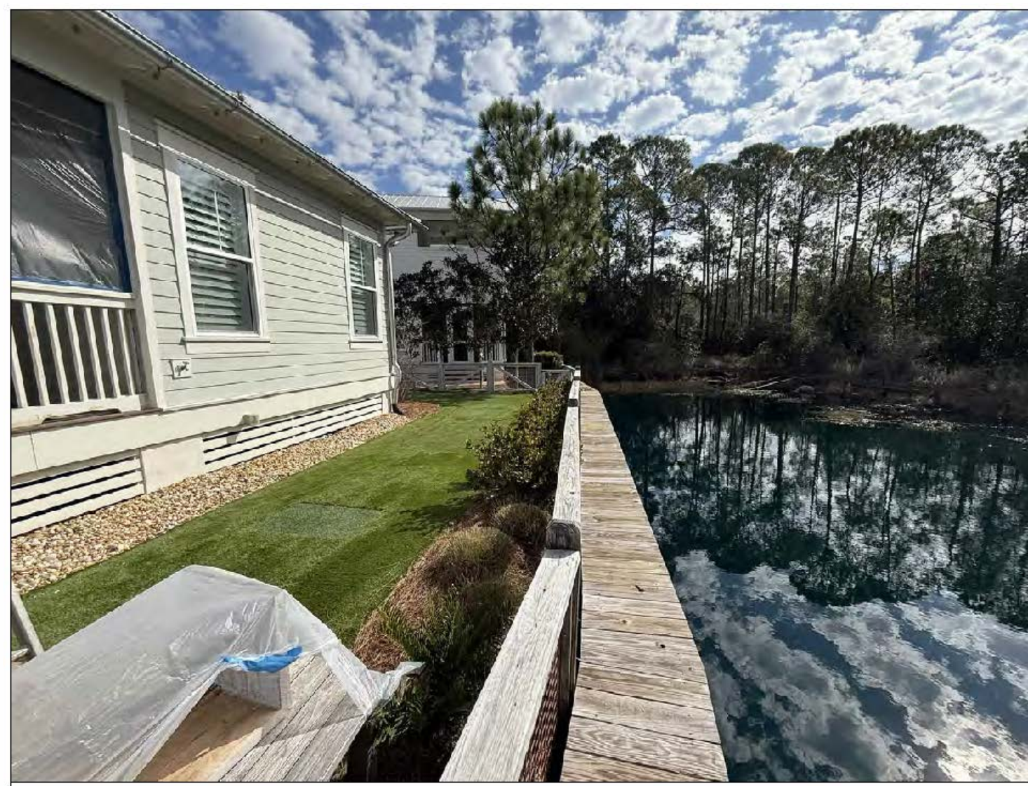
VEGETATION ENCROACHMENT ON LOT 90
