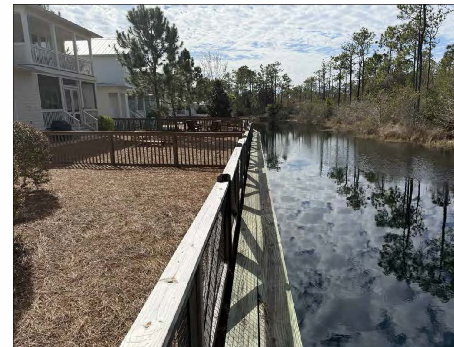
FENCE ENCROACHMENT BETWEEN LOTS 135 & 136
