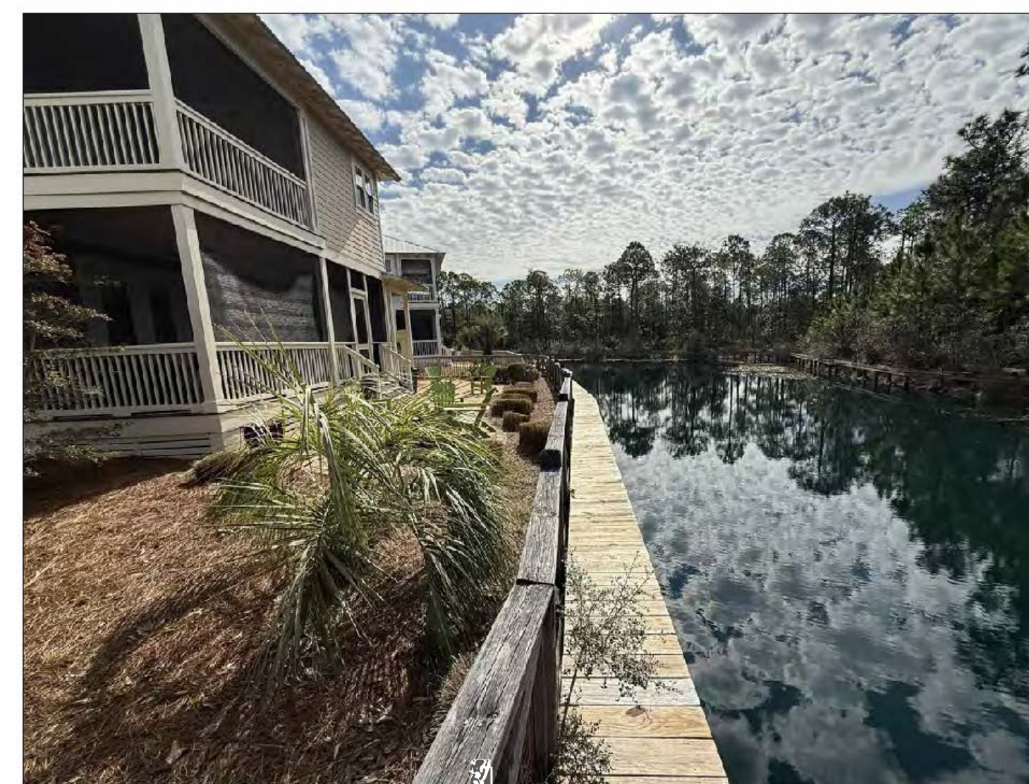
VEGETATION ENCROACHMENT ON LOT 88
