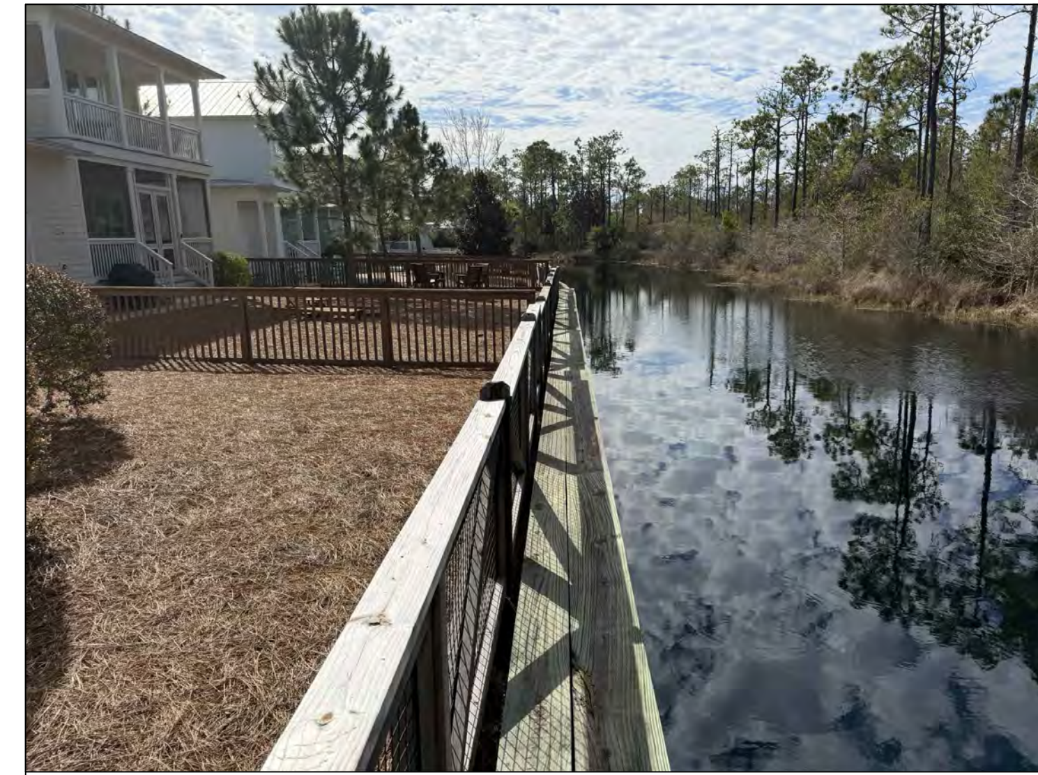
FENCE ENCROACHMENT BETWEEN LOTS 135 & 136
