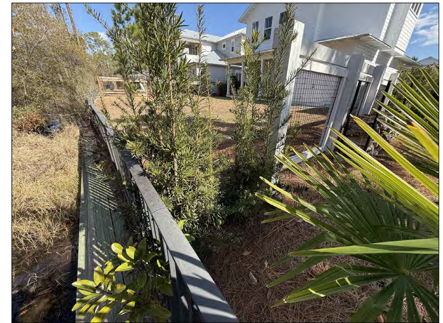
FENCE/VEG ENCROACHMENT BETWEEN LOTS 255 & 256
