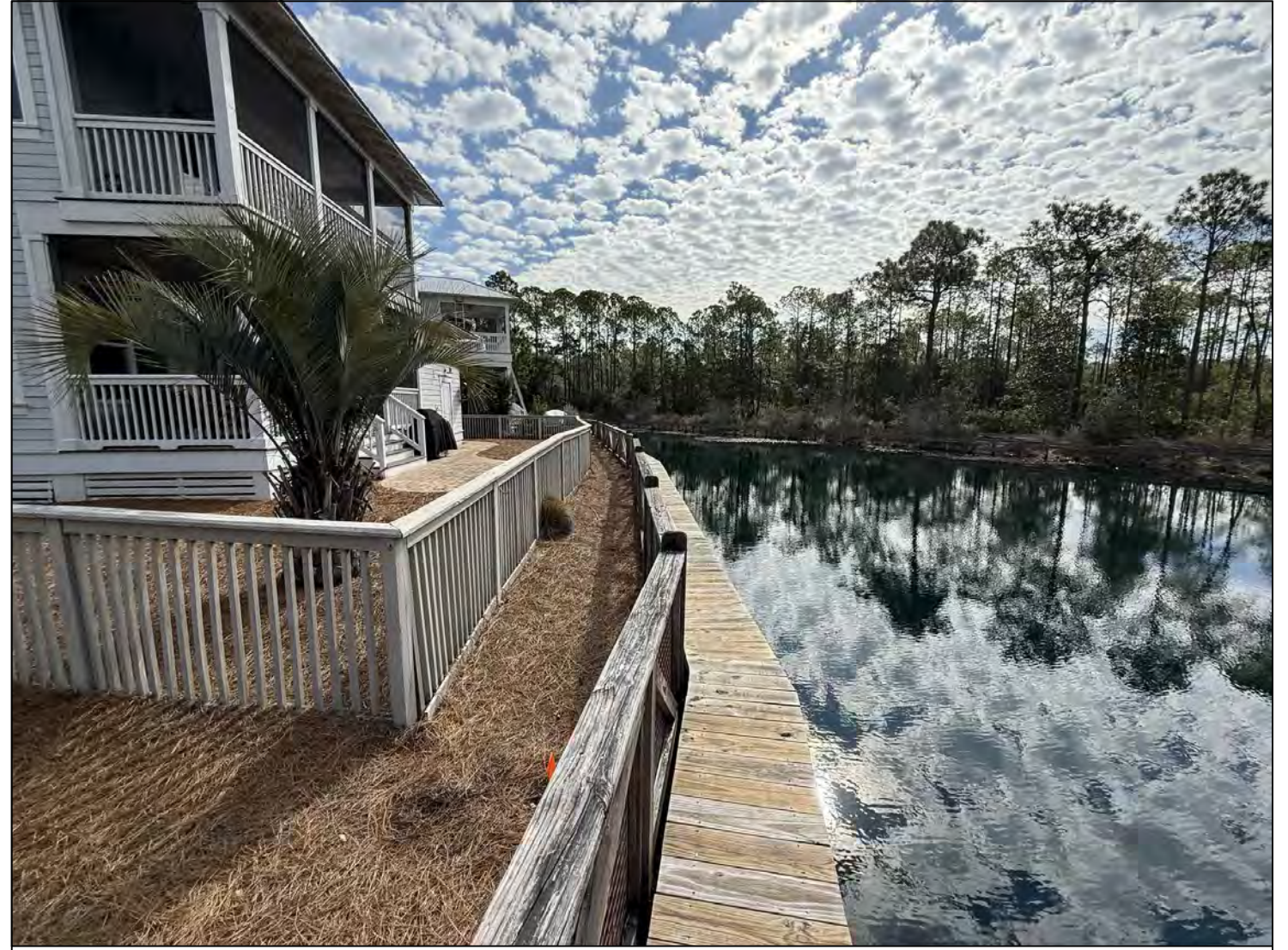
VEGETATION ENCROACHMENT ON LOT 89
