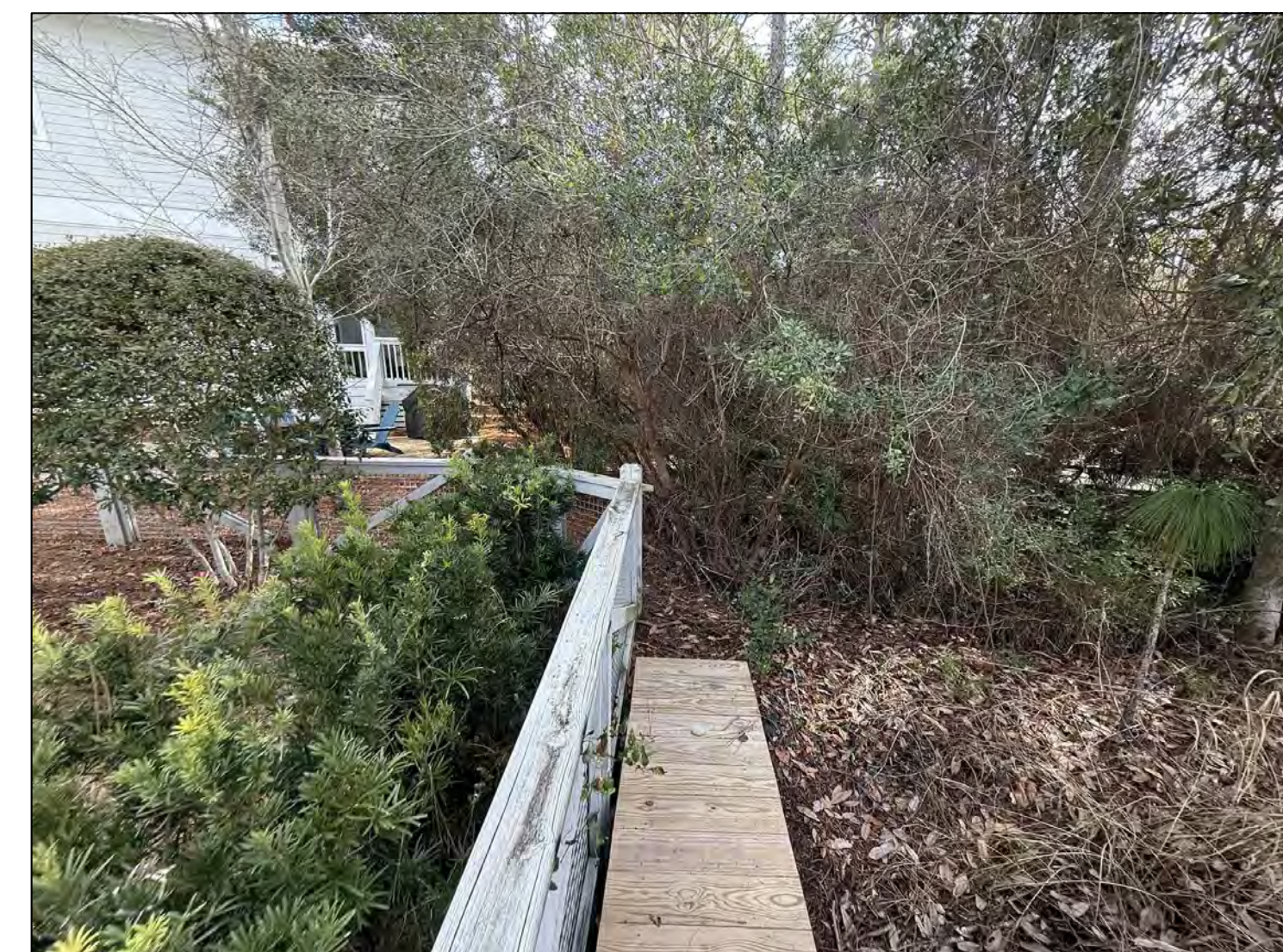
FENCE/VEGETATION ENCROACHMENT ON LOT 91
