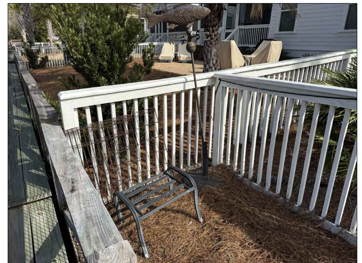
FENCE ENCROACHMENT BETWEEN LOTS 130 & 131
