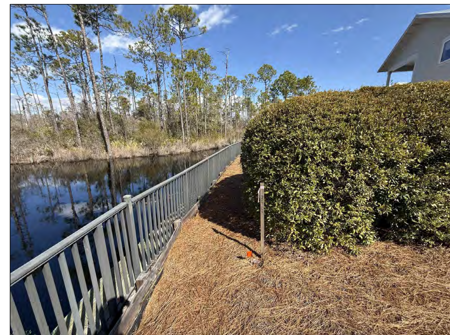
CDD FILL/WALL BEHIND LOT 259
