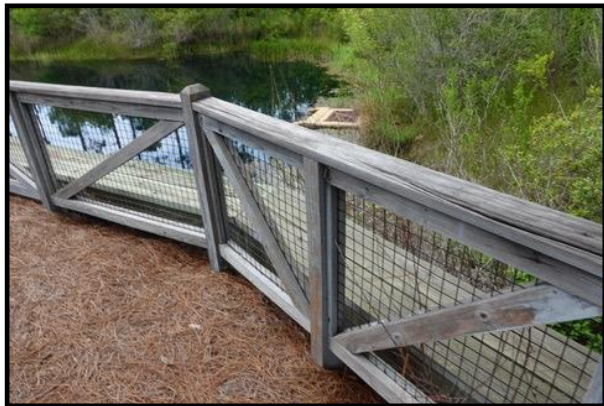
Figure 1 – Typical Bulkhead Railing
