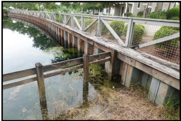
Figure 1 – Typical Vinyl Bulkhead with Wood Cap
