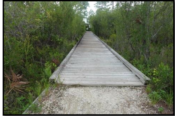
Figure 2 – Trail Walk Guardrails
