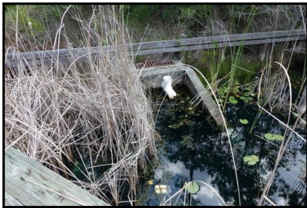
Figure 3 – Stormwater Pond Structure
