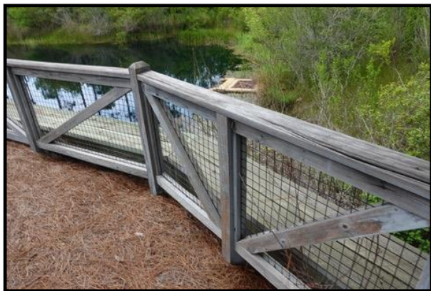
Figure 1 – Typical Bulkhead Railing
