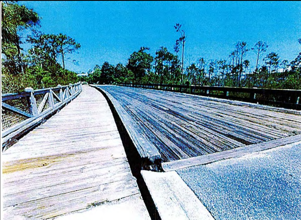
VIEW OF TYPICAL BRIDGE
