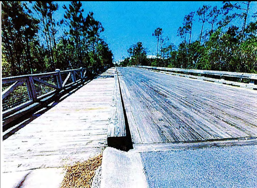
VIEW OF TYPICAL BRIDGE
